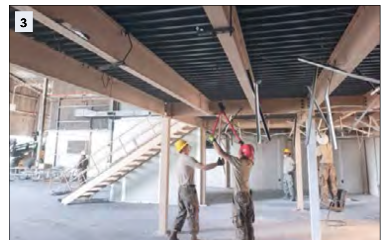
3) Crews from the 60th Civil Engineer Squadron structures shop dismantle old mobile offices July 2 inside Bldg. 844 at Travis Air Force Base. The refurbished hangar houses the new Nose Dock Gym. 4) New cushioned flooring covers the Nose Dock Gym Oct. 11 at Travis. 5) From left to right, Col. Victor Beeler, 60th Mission Support Group commander, Barbara Green, 60th Force Support Squadron programs director, Tanya McCormick, 60th FSS fitness and sports director, and Chief Master Sgt. Matthew Pulsipher, 60th MSG interim superintendent, stand inside the Nose Dock Gym Oct. 11 at Travis.
